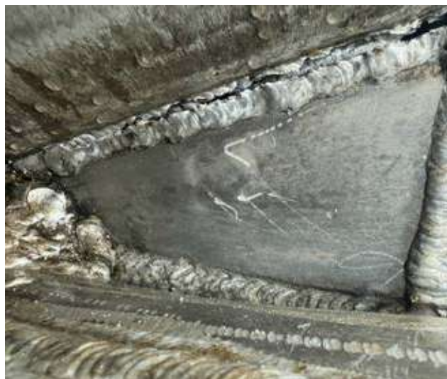
After having cleaned the bilge, a close look revealed broken weld seams.
